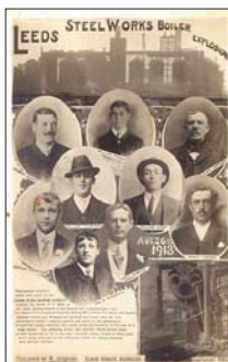
306. WARNER GOTHARD Leeds steelworks boiler ex- plosion. Surface creases but rare F.£40
