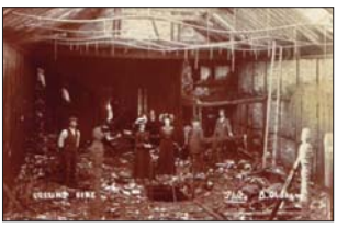
274. WISBECH fire at Collins' factory 1908 RP pub'd OldhamVG..£25
